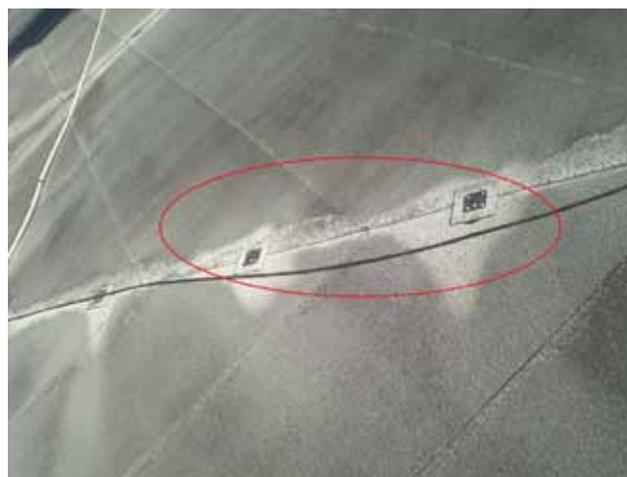
If there are skylights (see below), they should be checked for securement. Skylights that are not well sealed and secured around the frame's edge can leak, which may cause the skylights to become dislodged and allow for wind driven rain and debris to enter the building, especially during a high wind event.
