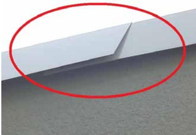
Tears in the roof cover (see below), or worn or cracking seams, can allow water to enter below the cover.
